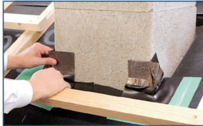
Inner corners plastering not possible
