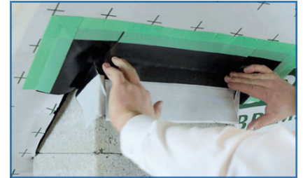
Inner corner can be plastered over
