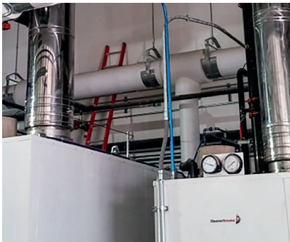
CONDENSING BOILERS
